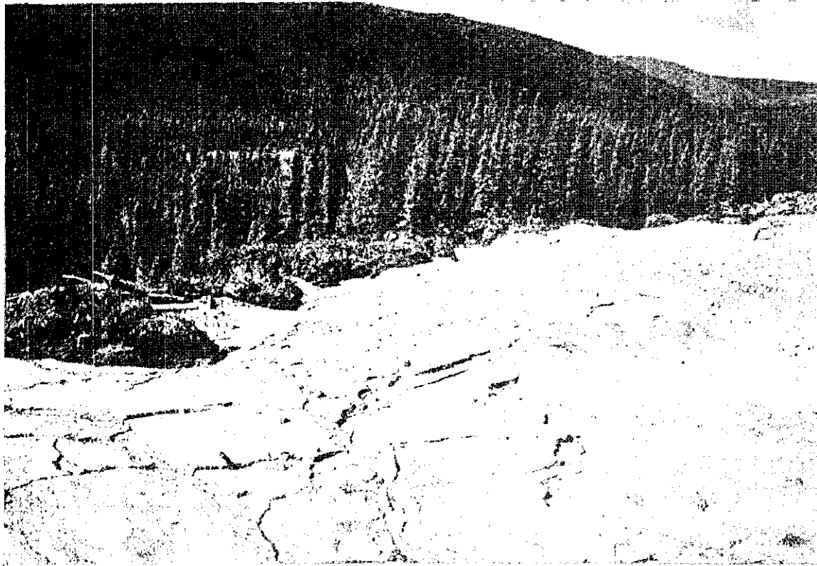
Solo Creek Dump Ice rich waste material from Water Supply Reservoir Dam Excavation July 1995
