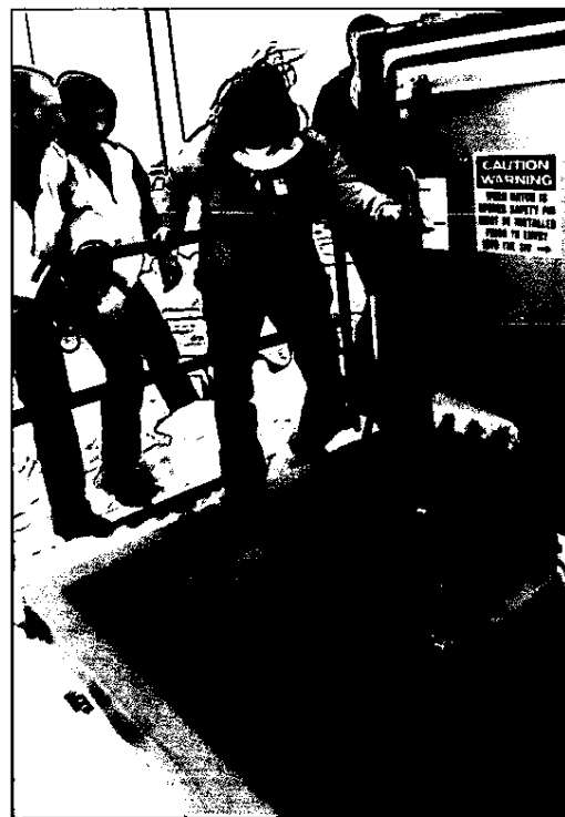
Windy Weather. Jamie Abordonado, ESGR executive director, holds on to the safety handle leading down into the silo interface vault on the Missile Defense Complex at Fort Greely. The ESGR group visited Fort Greely on an uncommonly windy day, with gusts reaching 70 mph.
