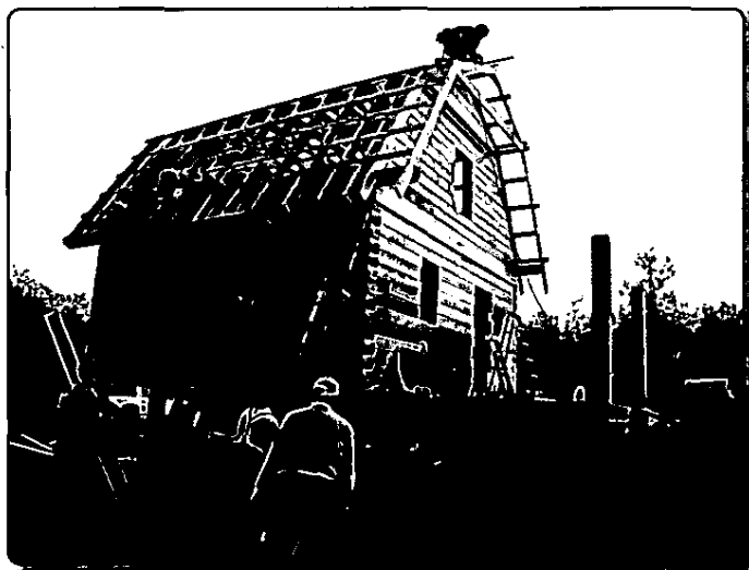
Rebuilding Mission. Mennonite volunteers finish the final cabin in Eagle 106 days after the housing mission began. The Disaster Housing Task Force played a major role in organizing and supporting more than 500 volunteers who contributed to the rebuilding effort. Photo: Courtesy of Roy Williams
