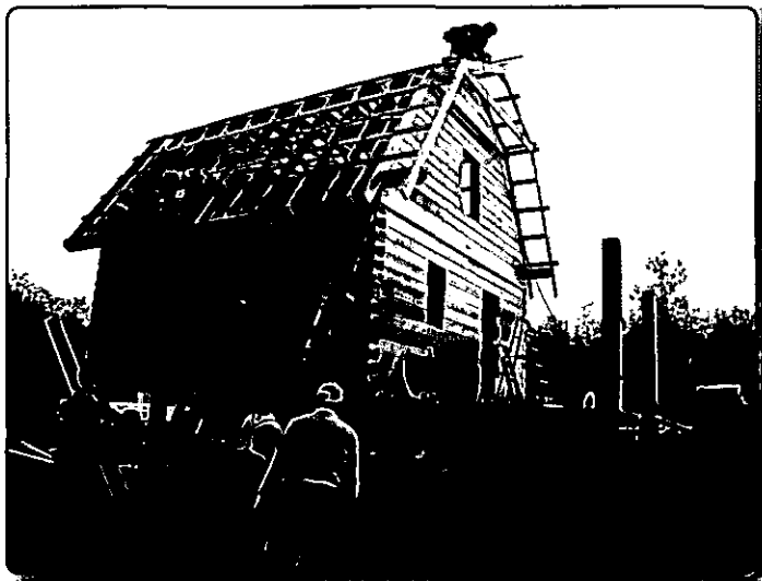
Rebuilding Mission. Mennonite volunteers finish the final cabin in Eagle 106 days after the housing mission began. The Disaster Housing Task Force played a major role in organizing and supporting more than 500 volunteers who contributed to the rebuilding effort. Photo: Courtesy of Roy Williams
