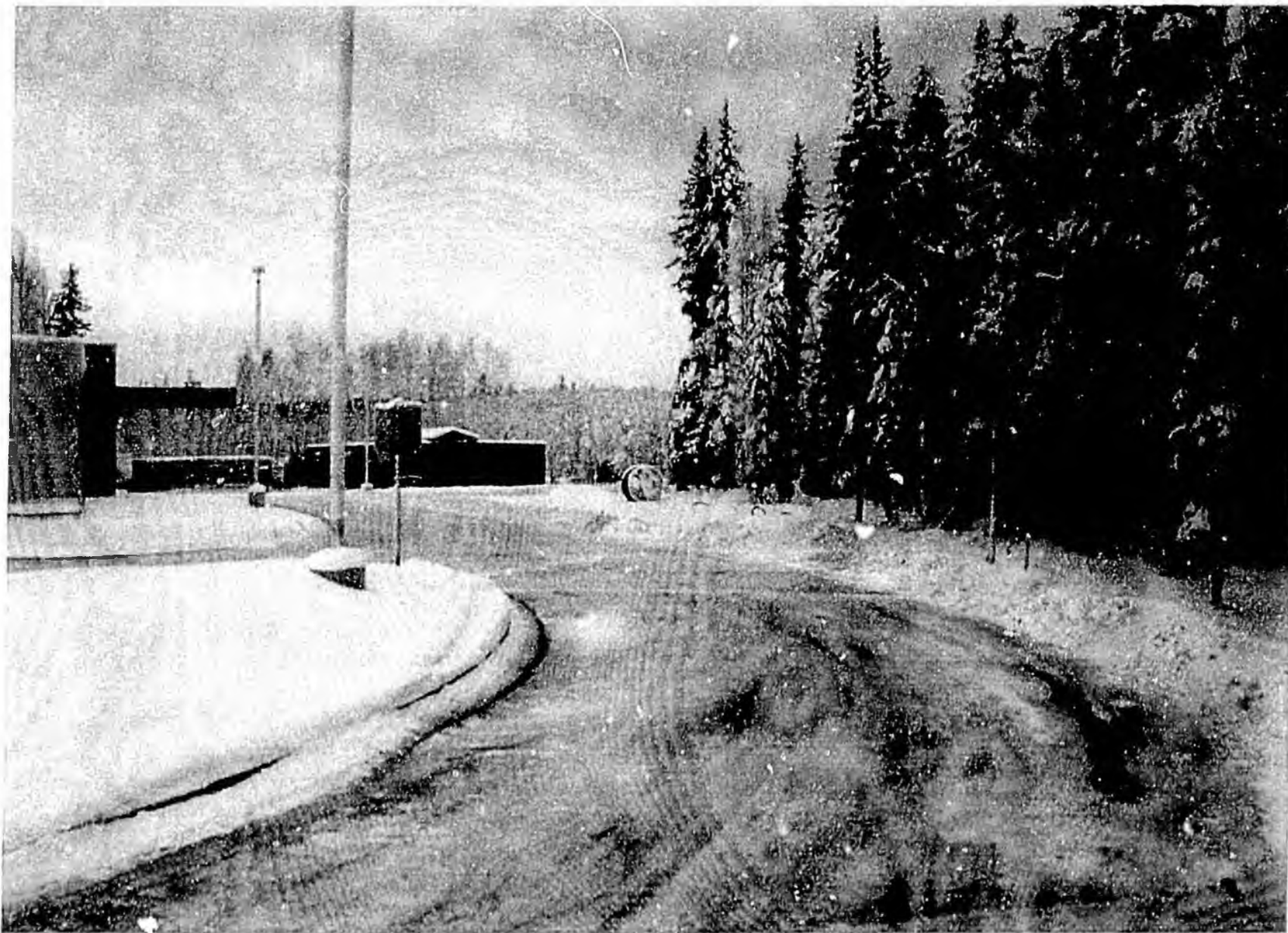
Proposed site of Virology Laboratory – Connects to BiRD Facility on left
