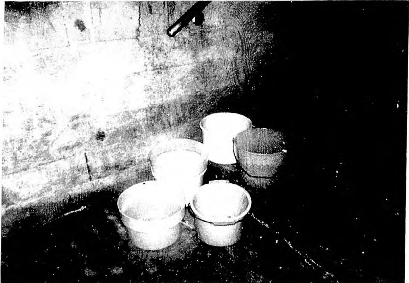
Existing roof leaks at Sitka Pioneer Home – North Wing
