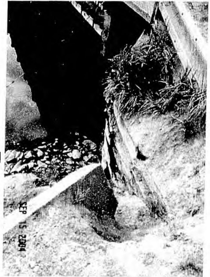
Damaged Piles from Ice Flows
