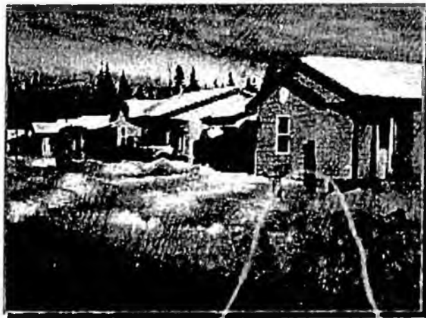
Mooring Estates, Soldotna FY1996
