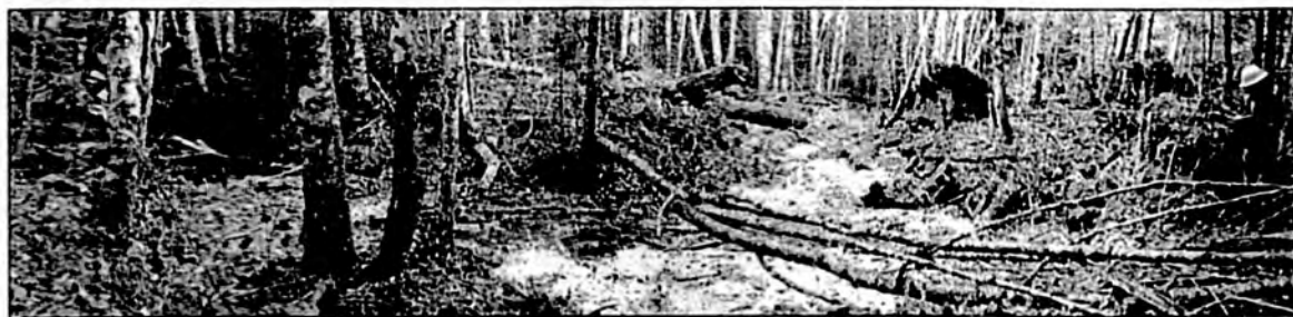
Same panoramic view 60 minutes after shot, most blasting debris stayed within a 40 foot radius, all fish in traps lived. TOP: view from downstream of flow through site immediately after shot. MIDDLE: flow through site 2 days later.
