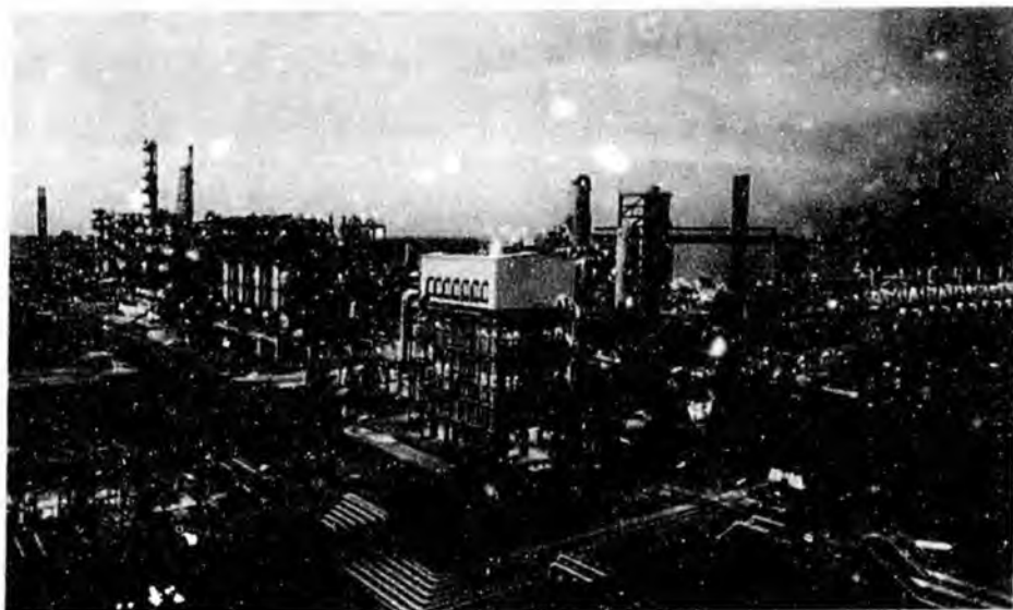
Shell Bintulu 15,000 BPD Gas to Liquids (GTL)
