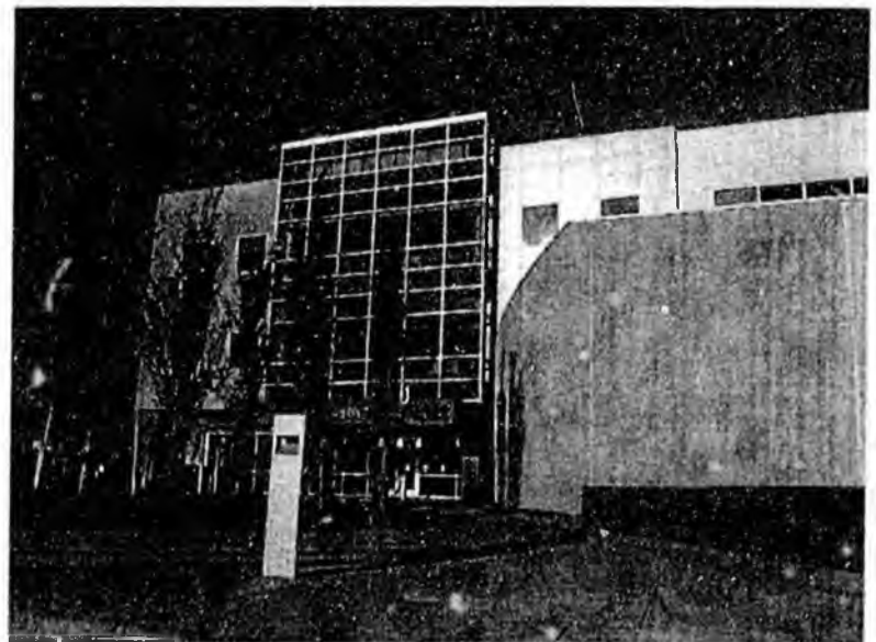
Orthopedic Physicians Building, Anchorage
