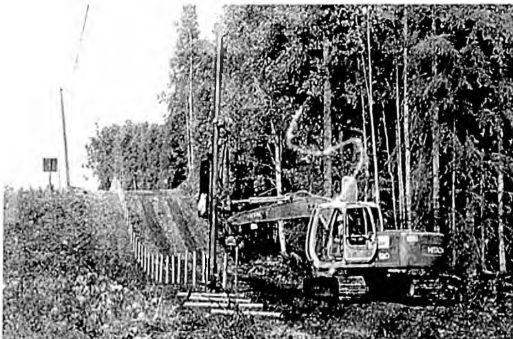
Fence Addition, Fort Richardson, Anchorage
