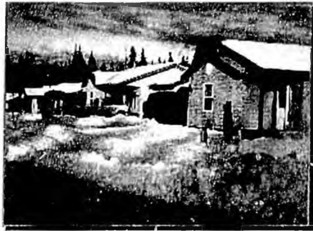
Mooring Estates, Soldotna FY1996
