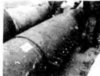
Line leak and sleeve installation
