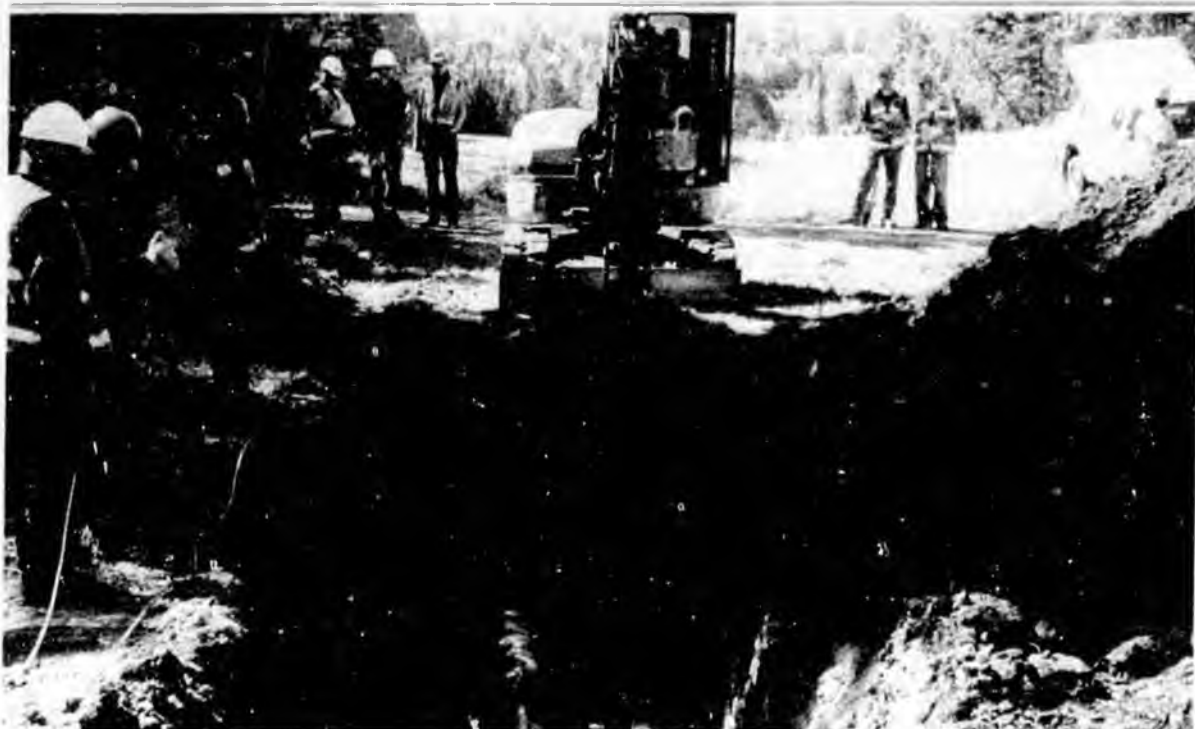
In July, 2005, the compliance oversight team observed a pipeline integrity dig at a potential external wall loss location identified in an in-line inspection run. No anomaly was found.
