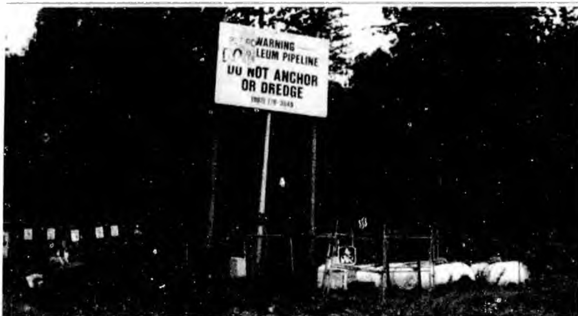
This sign, a piece of which has fallen off, marks the pipeline's transition to sub-sea at Point Possession on the Kenai Peninsula. The propane tanks to the right are part of the impressed current cathodic protection system for the sub-sea line. The site was accessed by four-wheeler during June 2006 SPCO surveillance.
