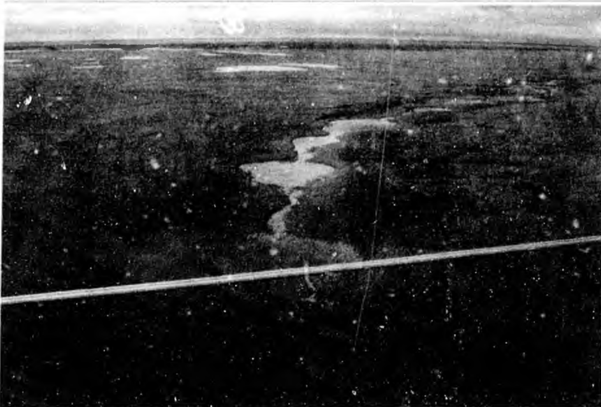
The Alpine Pipelines (oil, diesel, and utility) connect the Alpine Development on the Western North Slope to infrastructure in the Kuparuk River Unit.
