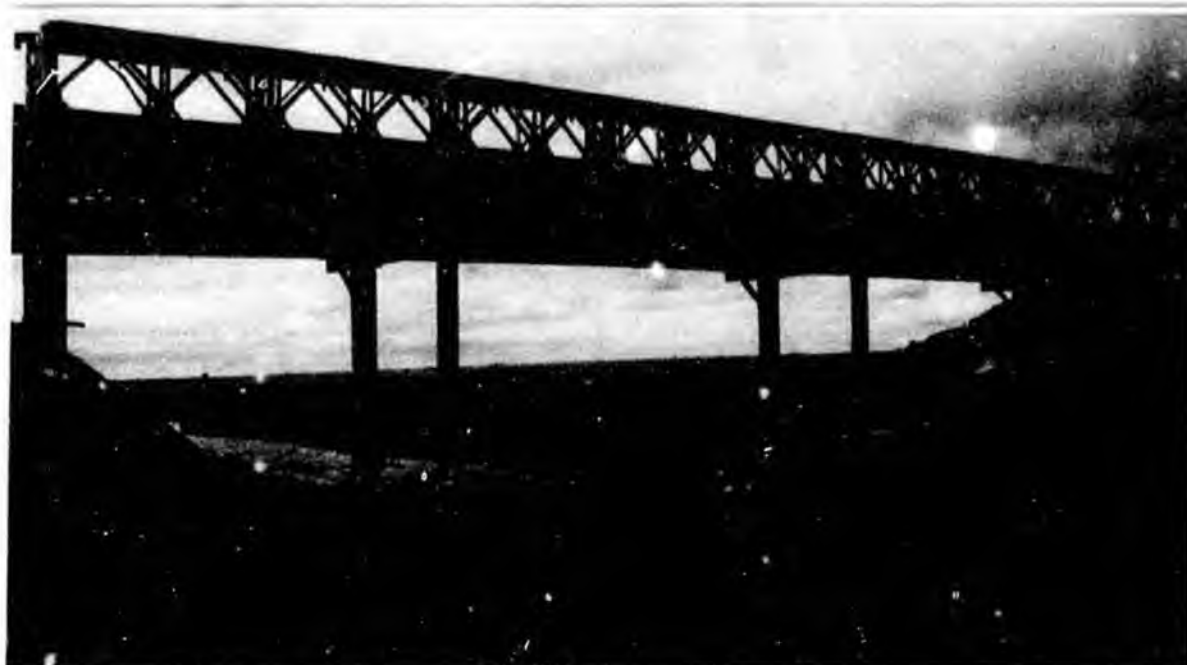
The KPL and OPL cross over Smith Creek, a Kuparuk River tributary, on the Bailey Bridge. CPAI also maintains the Hamilton Bridge as part of the KPL/OPL access road.
