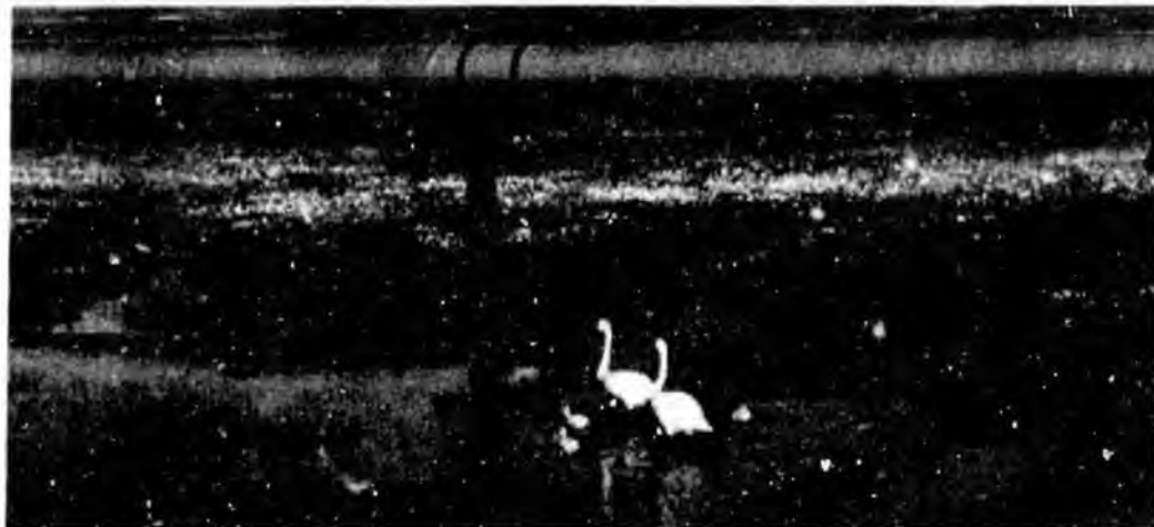
The Endicott Pipeline passes through important tundra and wetland habitats. Here a pair of swans and their three young are using wetlands next to the pipeline. The smaller pipeline in front is the Badami Utility Pipeline, which is on the same supports as the Endicott Pipeline from Endicott to the Badami/Endicott tie-in.
