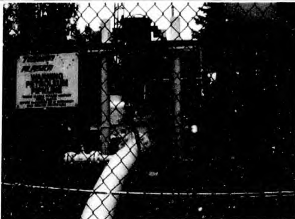
This photo is of a remotely-operated valve on the Nikiski Alaska Pipeline near Point Possession. Solar panels and propane provide energy for the valve and cathodic protection system.
