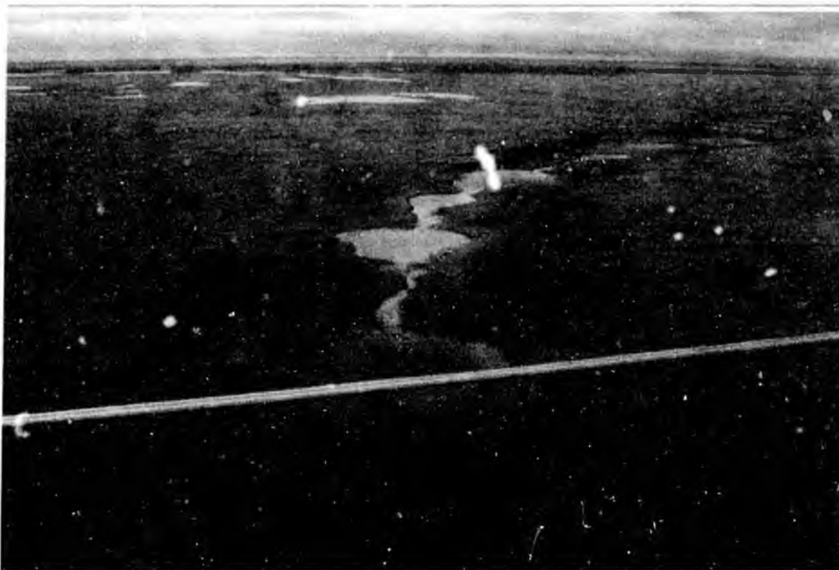
The Alpine Pipelines (oil, diesel, and utility) connect the Alpine Development on the Western North Slope to infrastructure in the Kuparuk River Unit.
