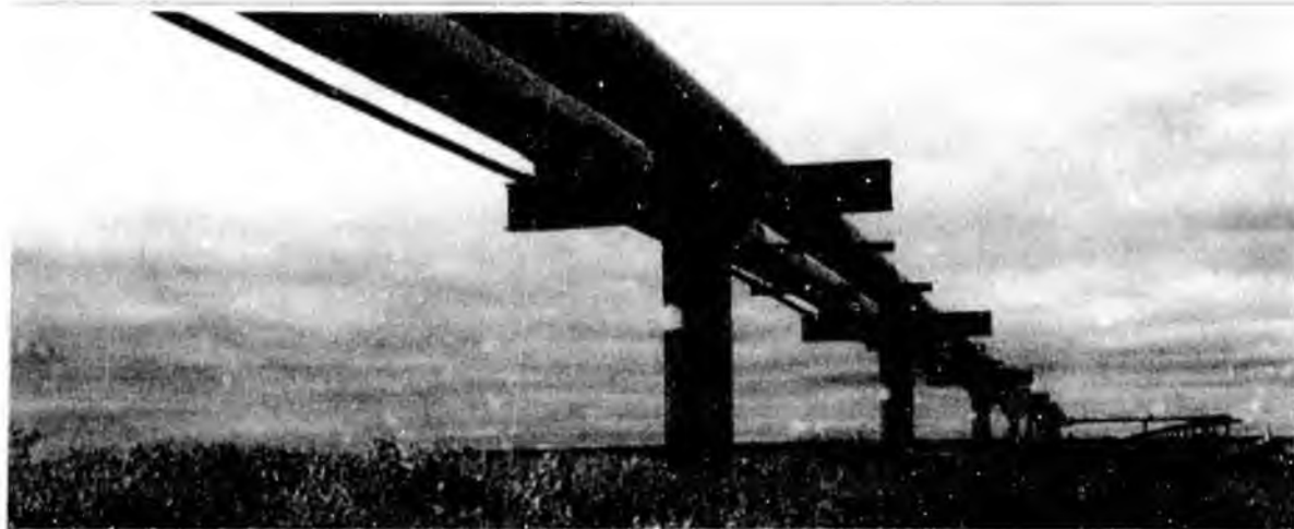
VSMs for the Alpine pipelines are marked with reflector tape for public safety.
