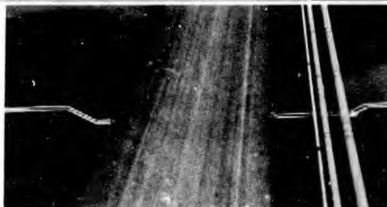
At road crossings, the Northstar pipelines are located in steel culverts covered with gravel. This picture was taken from a helicopter during an SPCO compliance oversight visit in 2004.
