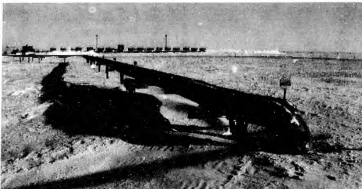
View of the Milne Point Pipelines looking east from Milne Point Road. The pipelines transition to a buried road crossing. In the background is Milne Central Facilities Pad.
