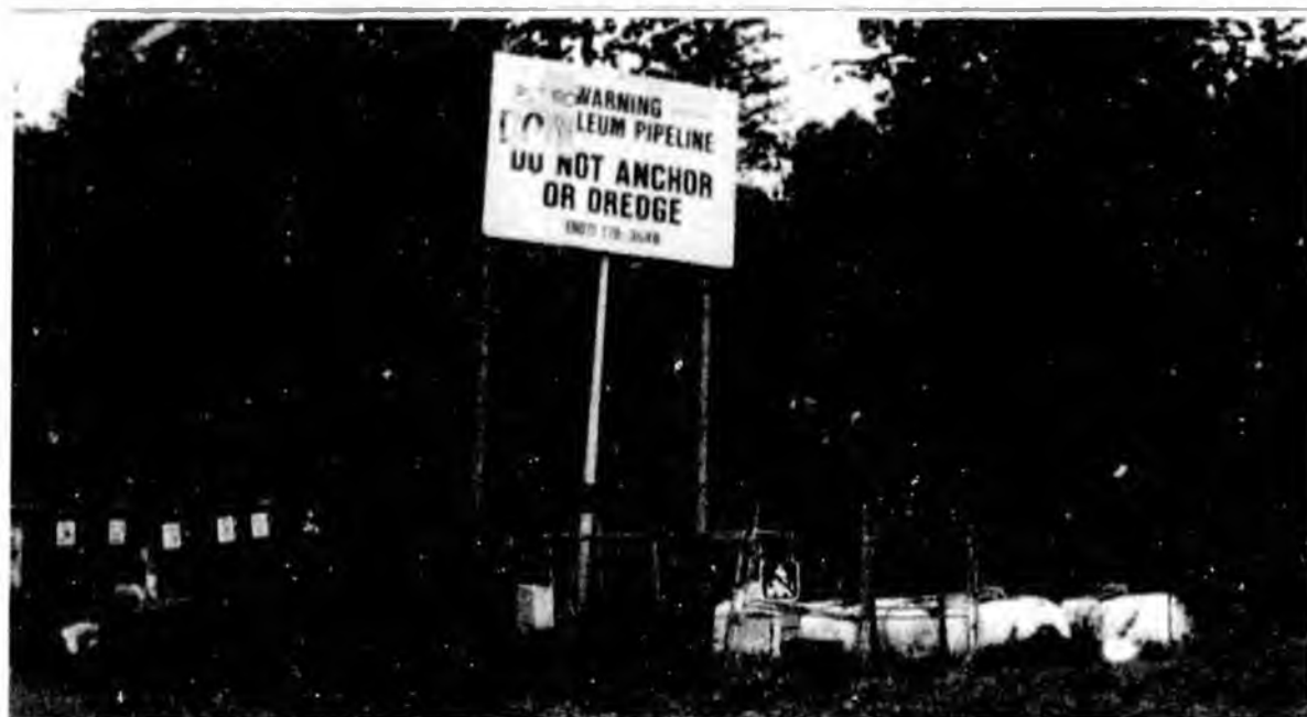
This sign, a piece of which has fallen off, marks the pipeline's transition to sub-sea at Point Possession on the Kenai Peninsula. The propane tanks to the right are part of the impressed current cathodic protection system for the sub-sea line. The site was accessed by four-wheeler during June 2006 SPCO surveillance.
