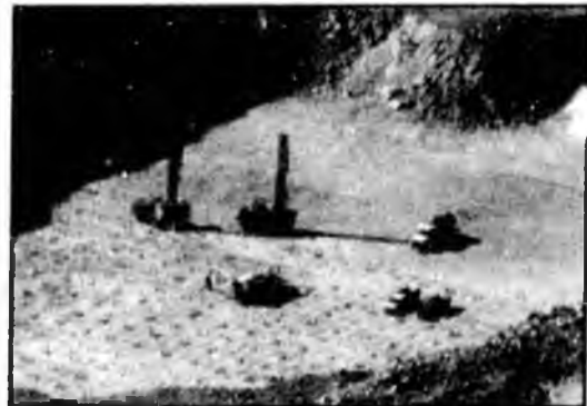
Holes are drilled and filled with explosives prior to blasting.
