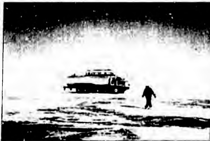
Figure 4: Ice road construction begins when the active layer is satisfactorily frozen. Snow is packed and then pumped water is sprayed onto the snow surface until a sufficient road thickness is attained (photo — W. Morris).
