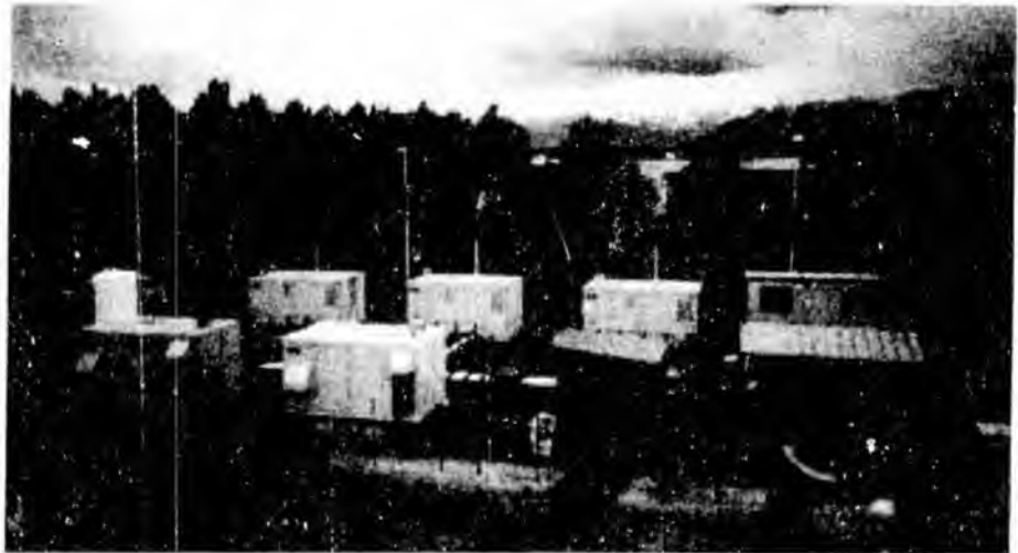
Set against the Chugach Mountains, five fuel cells supply reliable and clean power to the USPS facility.
