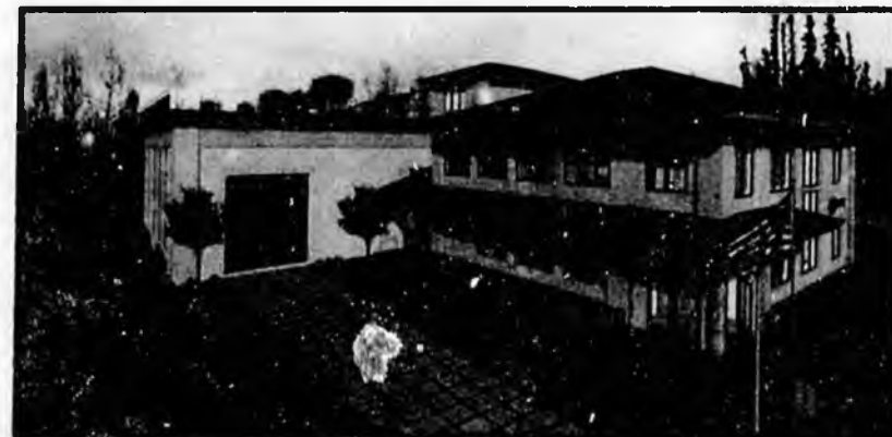
Cold Climate Research Test Facility
