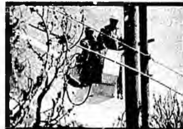
In August 2002, SDG&E workers battled difficult conditions to replace power poles and other equipment damaged in a fire that burned more than 60,000 acres in eastern San Diego County.
