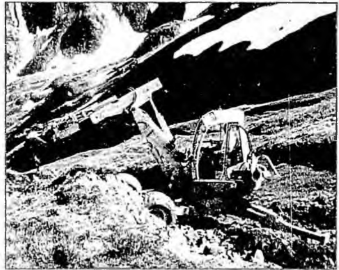
A "Menzi muck" machine carries out a trench to bury power lines. Photo is courtesy of Alaska Electric Light & Power Company.
