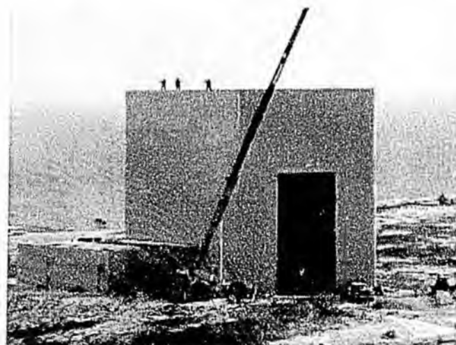
Payload Processing Facility (PPF)
