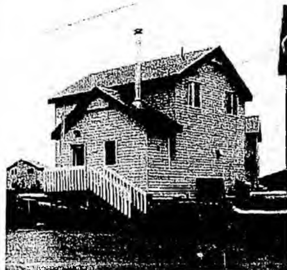
The Public Housing Division owns and operates several hundred single family homes throughout Alaska, like this weathered home in Bethel.
