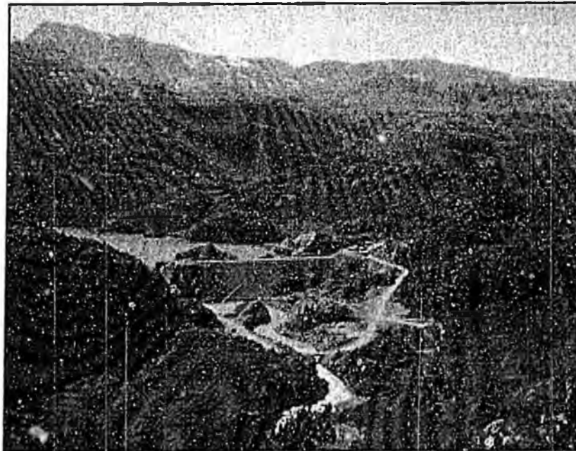
Bradley Lake Hydroelectric Project
