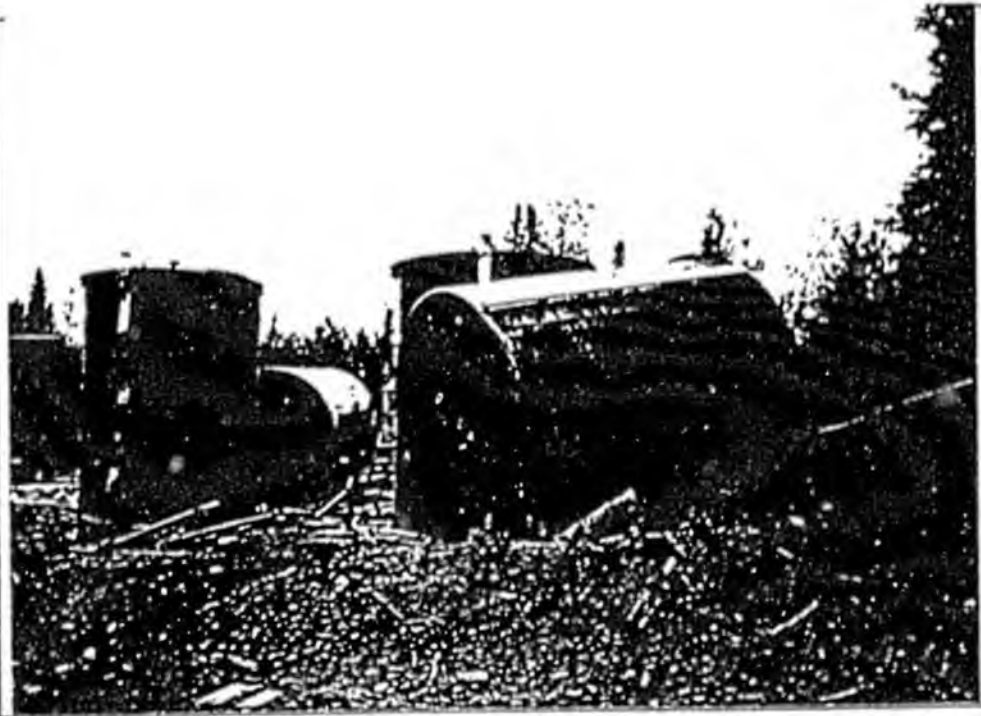
Photograph A.13 Tank farm located within a flood plain. Tanks tipped over and facility severely damaged by flood.
