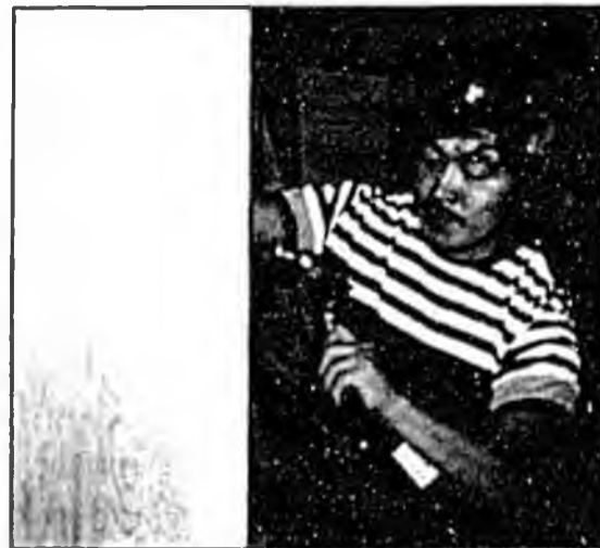
Enoch Porter works on the utility shed in Kotzebue.
