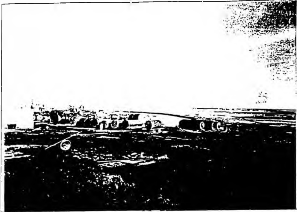
Photograph A.5 Tanks scattered along river bank with no dikes, no security, and improper foundations.
