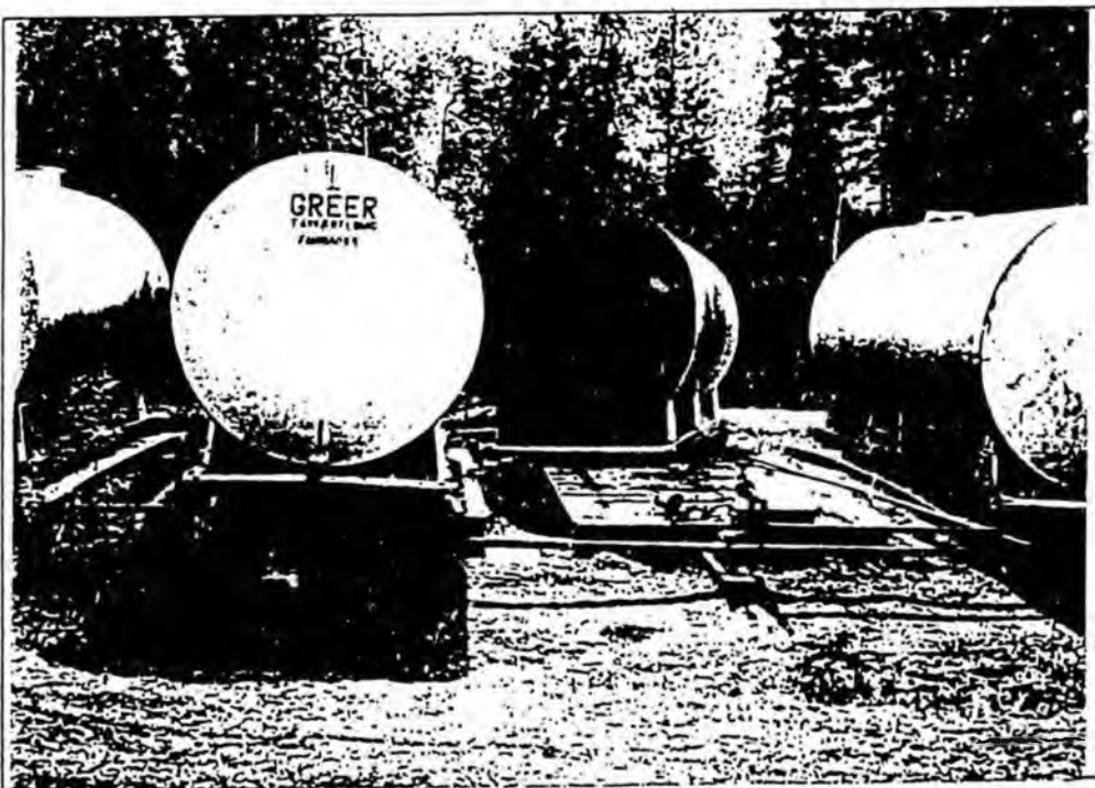
Photograph A.8 Improper piping system and poor operational procedures resulted in explosion of tank.
