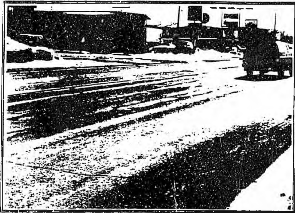
Studs have worn through the top pavement layer ( 2'' \pm ) along lines spaced equally with car wheels.
