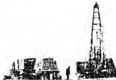
Figure 3. Winter drilling operations at Deadfall Syncline.
