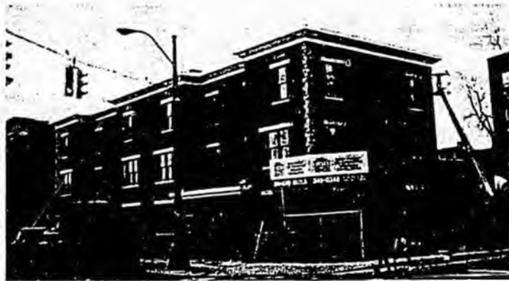
Eight families invested 2,750 hours of “sweat equity” to renovate this building in Hartford, Conn., where they are now proud first-time homeowners in La Esquina Brillante.
