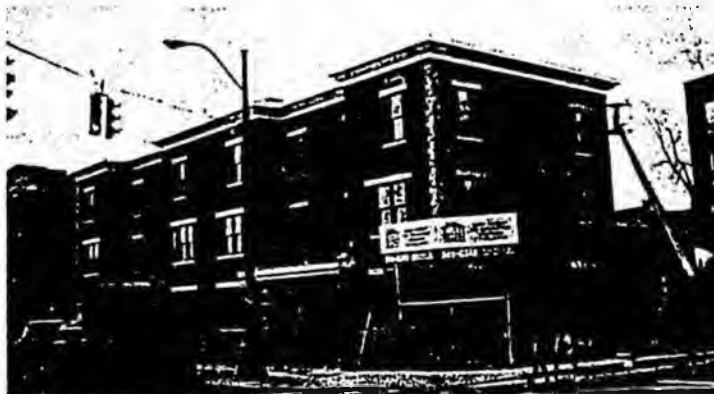
Eight families invested 2,750 hours of “sweat equity” to renovate this building in Hartford, Conn., where they are now proud first-time homeowners in La Esquina Brillante.
