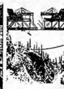
Washington State Historical Society Men build a railroad bridge across the Kuskulana River in 1910. Today travelers on the road to McCarthy cross this bridge.
