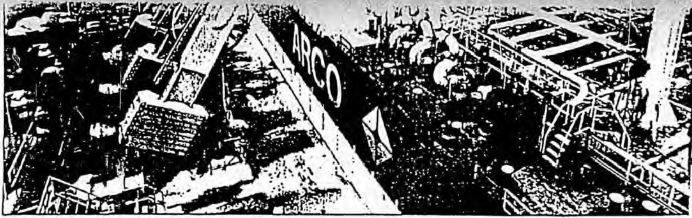
Three huge booms load an Arco tanker at the rate of 95,000 barrels of oil an hour at the Alyeska Port Facility in Valdez.
