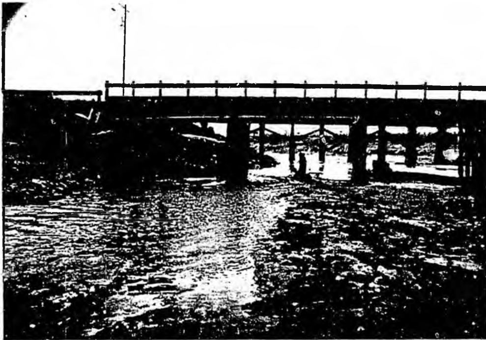
SOUTH END OF BRIDGE. NOTE WATER FLOWS TOWARD ABUTMENT.
