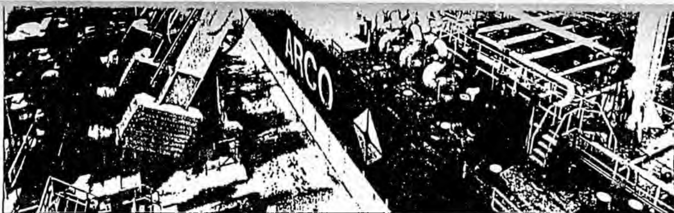
Three huge booms load an Arco tanker at the rate of 85,000 barrels of oil an hour at the Alyeska Port Facility in Valdez.
