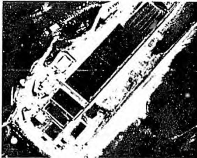
"Aerial view of leach pads and metallurgical plant"
