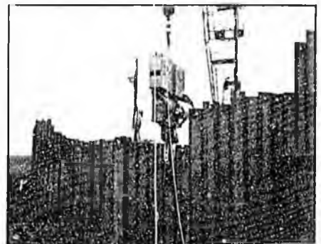
Up to 44,000 sq. ft. of sheet pile will be driven to form open-ended cells and flank walls at the abutments of four bridges. The design provides high load-bearing qualities while preventing fill encroachment into streams. PN&D photo.
