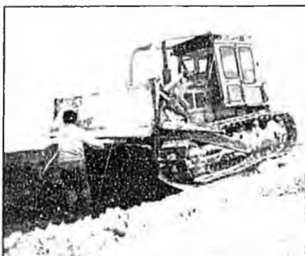
More than 1.1 million cu. yd. of geotextile was placed under the mine road, material site access roads and at bridge abutments. It was rolled out directly onto the tundra by ATVs in summer and with dozers after freeze-up. PN&D photo.
