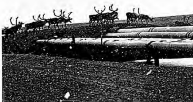
Although caribou use gravel ramps over pipelines at Prudhoe, studies have shown the ramps are not necessary.
