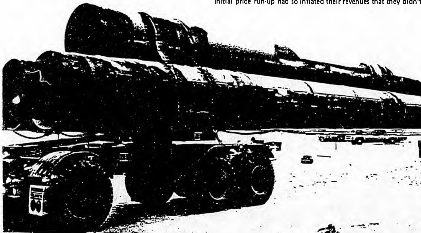
These sections of pipe were being moved from storage yards at Fairbanks, Valdez and Prudhoe Bay to intermediate storage sites along the 800-mile trans-Alaska pipeline route. (All pipeline photographs courtesy of Alyeska Pipeline Service Company.)
