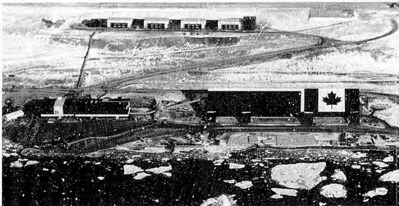
Above left: The swimming pool at Polaris is the most northerly in the world. Above right: The accommodation complex is raised off the ground so that heat transfer from the buildings does not melt the permafrost. Below: Aerial view showing the accommodation complex at the top, the concentrator (barge) at lower left and the storage shed (with maple leaf) at lower right.
