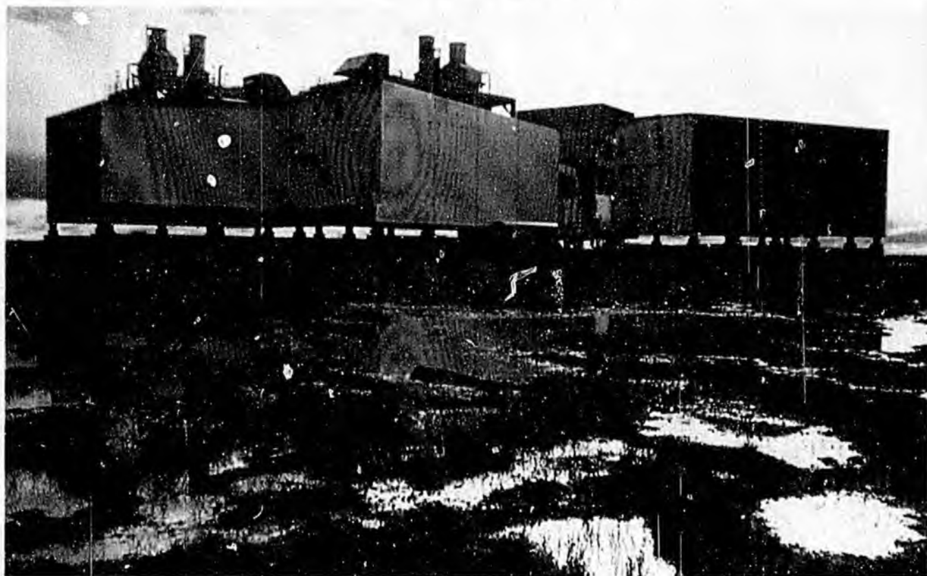
Modules for processing crude oil are seen at a module staging area at Prudhoe Bay on the North Slope of Alaska. They were built in Seattle.
