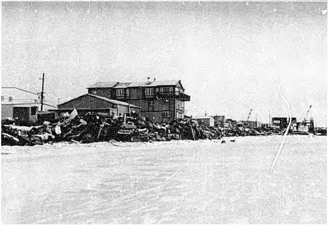
City business section of waterfront as seen from river. View is upstream toward cargo dock. Buildings in left foreground are part of ELM Fisheries. Note attempts to prevent loss of riverbank through the use of junked vehicles and other debris.
