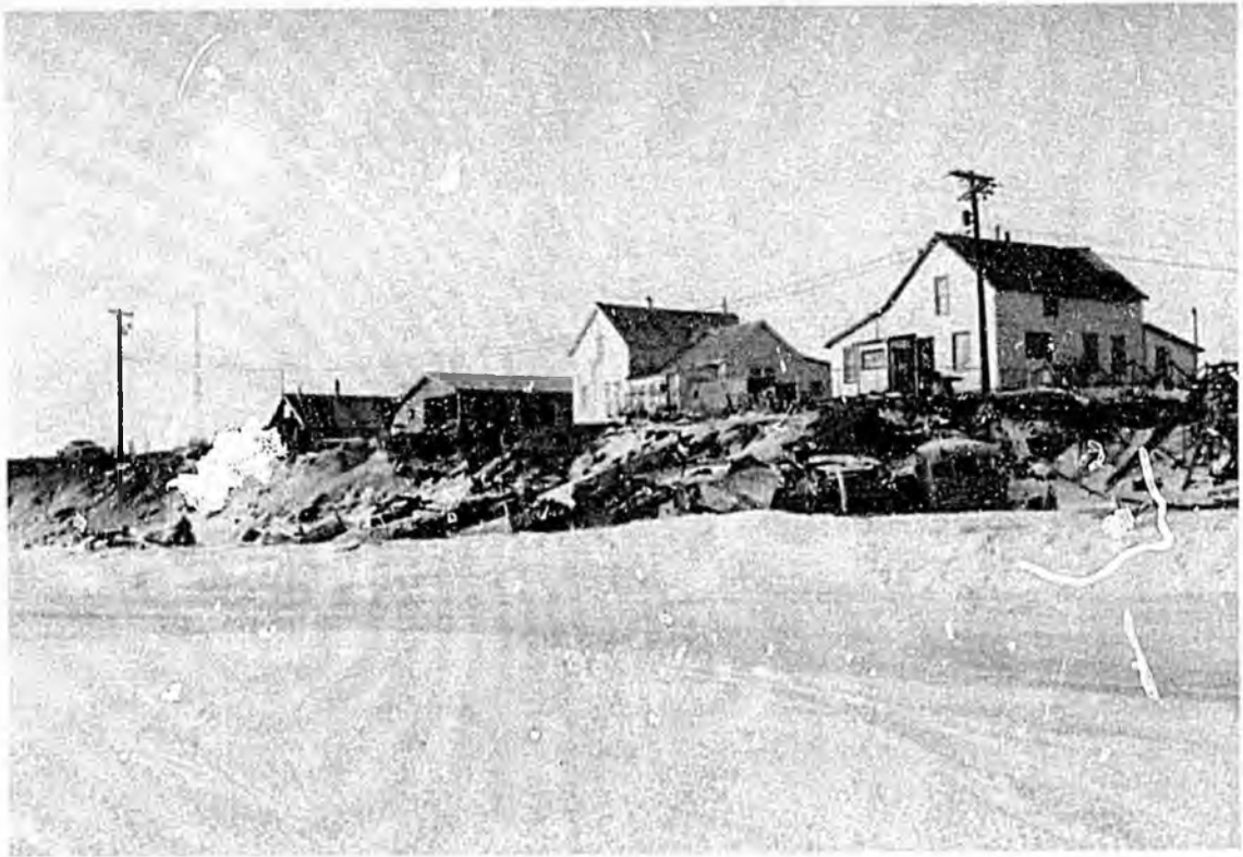
Mission Road area, looking downstream. Road has disappeared and houses are now at edge of riverbank.
