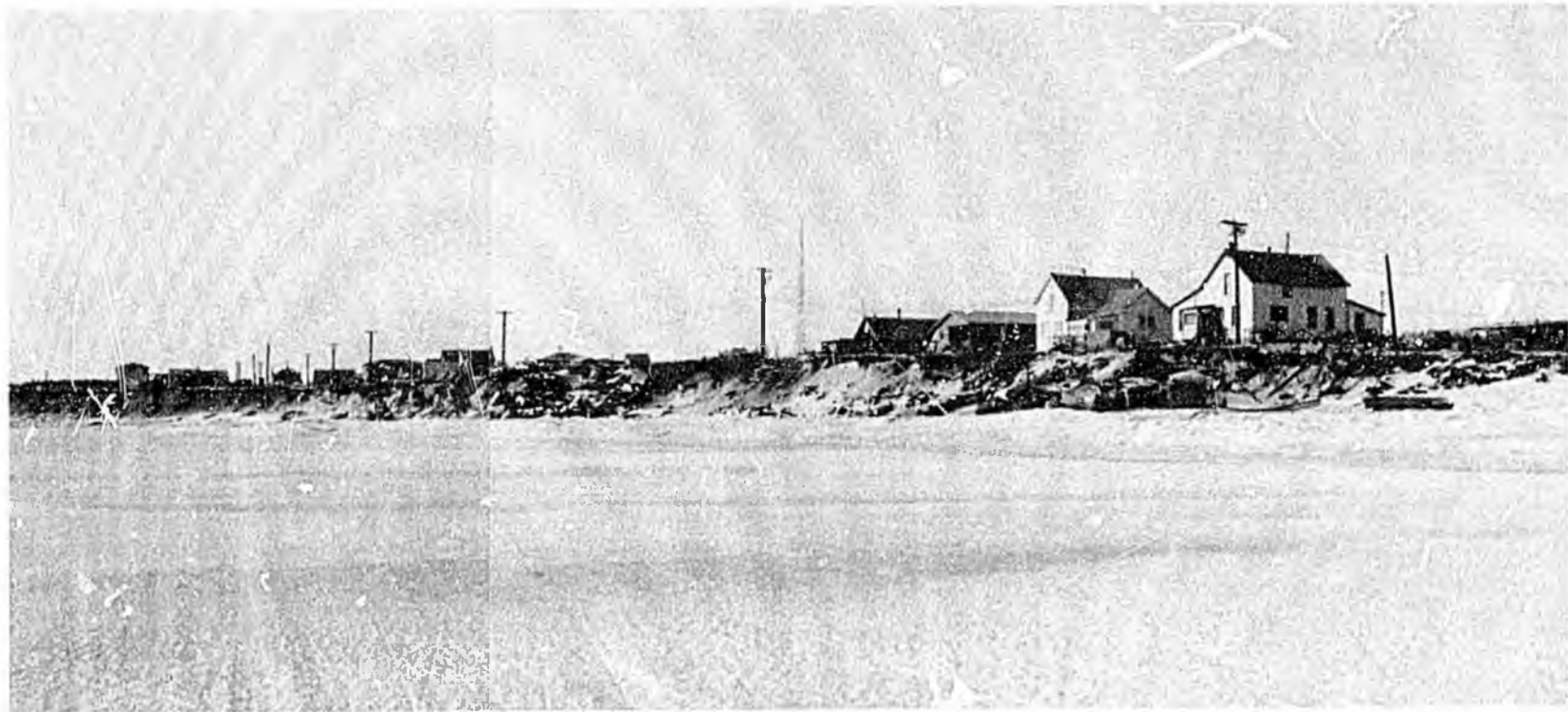
Mission Road area looking downstream. The road is now gone and buildings are at edge of riverbank. Note attempts to arrest loss of bank by using junked vehicles and other debris in same manner as at business section of the city.
