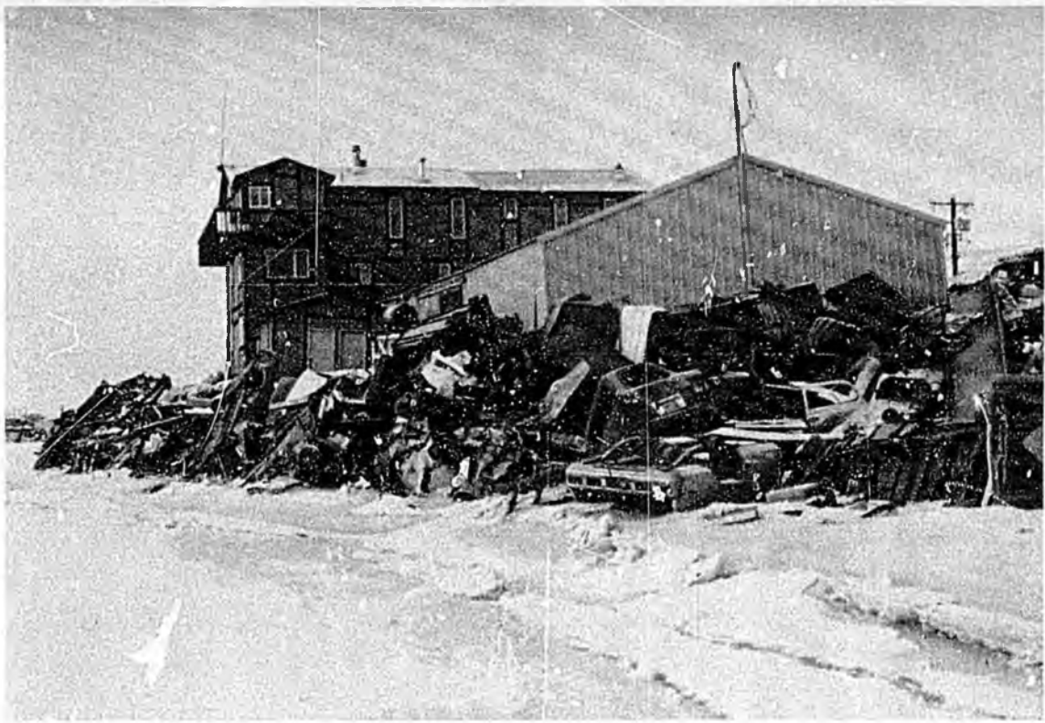
Close up view at attempt to arrest loss of riverbank at ELM Fisheries.
