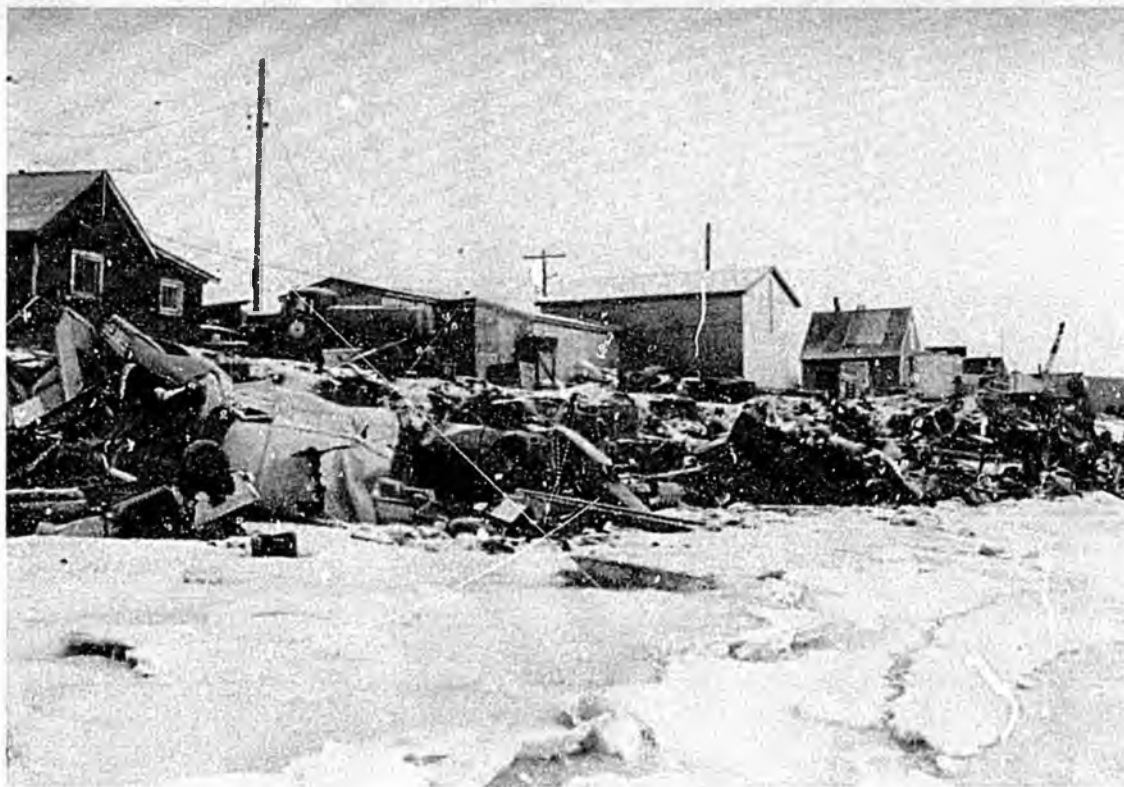
Closer view of riverbank erosion abatement measures currently in force at Industrial/Business section between ELM Fisheries and Cargo Dock. Looking upstream. See previous photos.
