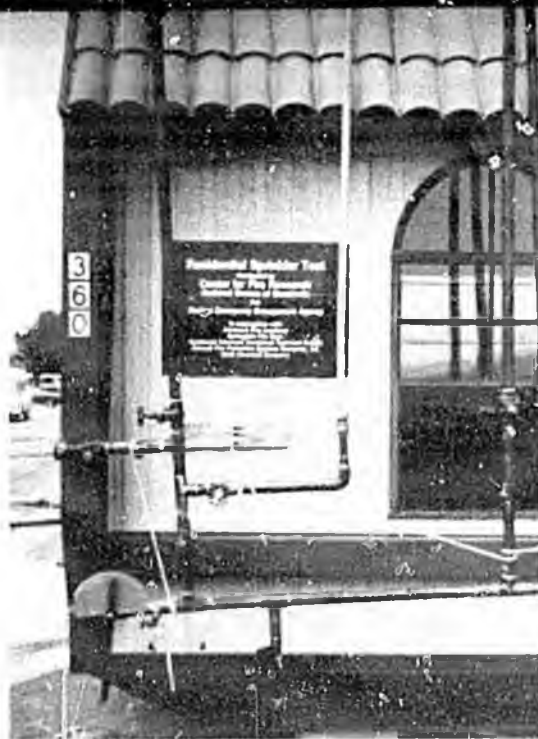
The Duralflex polybutylene line was attached to the existing water supply lines and ran below the roof.
