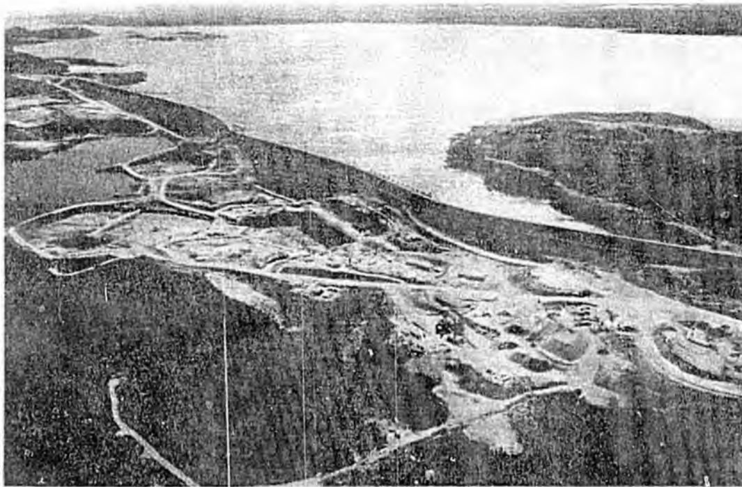
The LG 3 reservoir as it looks when it is partially filled: the main dam, spillway and powerhouse.
