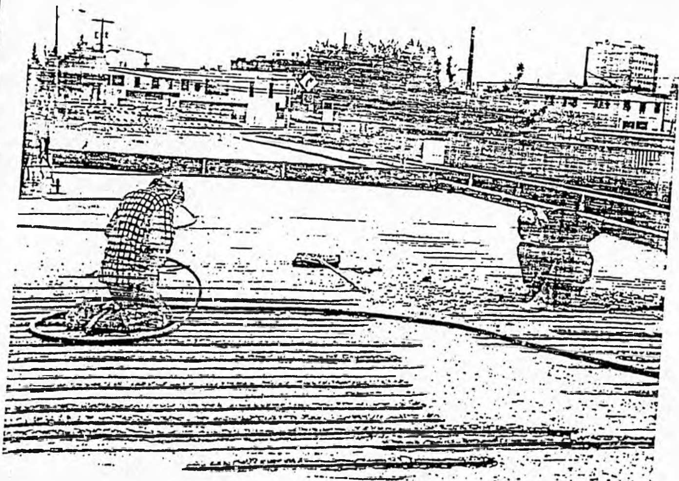
FIGURE 1 Removing delaminated concrete, Wendell St. Bridge, Fairbanks
