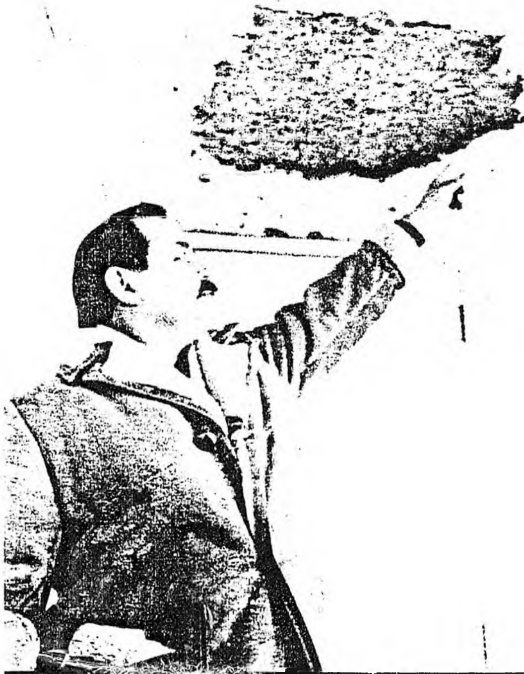
Asbestos hazards have been identified in thirteen Borough schools
