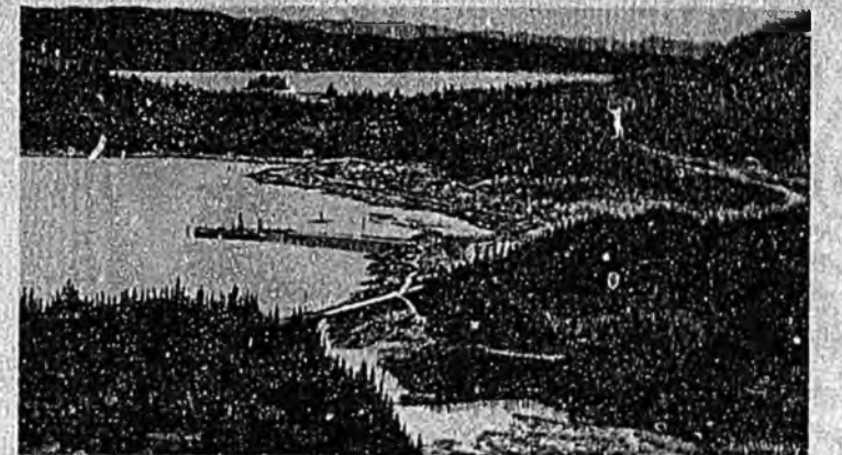
KP 10 Floating construction camp for construction workers at Ward Cove - June 30, 1952.
