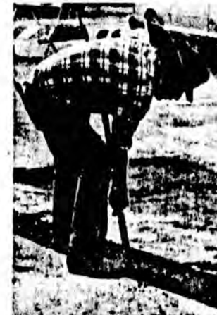
Art Hunter digs ground for Acme Electric of Fairbanks. His effort will modernize Fairbanks International Airport.
