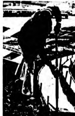
This cement form gets its final touches from John Jackson of Plasterers and Cement Masons Local 867.
