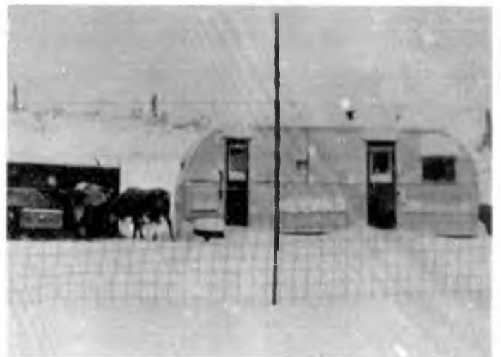
Food storage building (right) and "self-feeder" (left) within the main grazing paddock.
