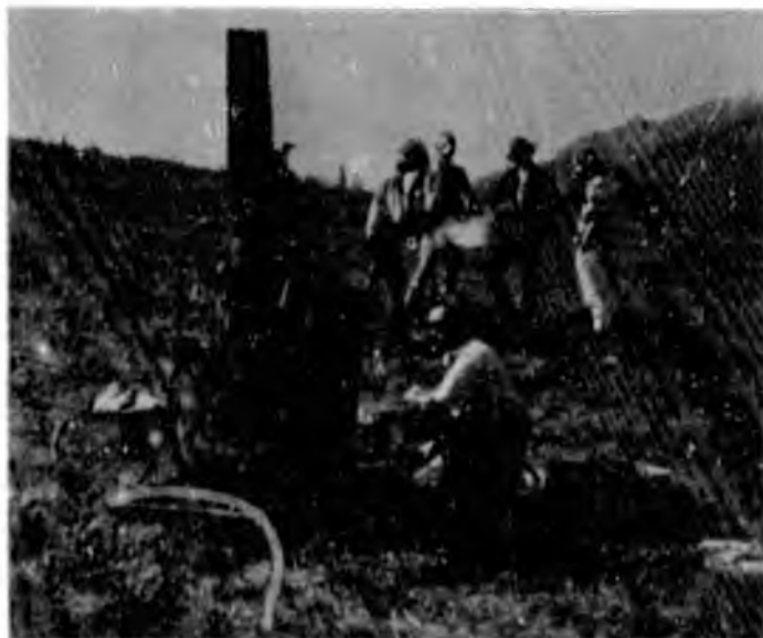
This photograph shows Cantwell resident Mike Pedro operating a steam jenny to thaw holes in the permafrost for fence posts.
