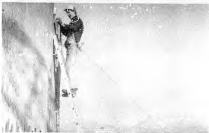
High above the street level, this apprentice is receiving valuable on the job training on a high rise building.
