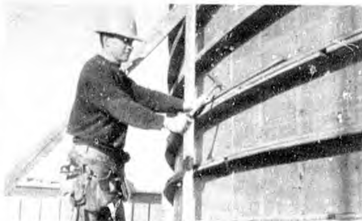
Securing this large circular form in preparation for a concrete pour is part of a day's work for this apprentice.
