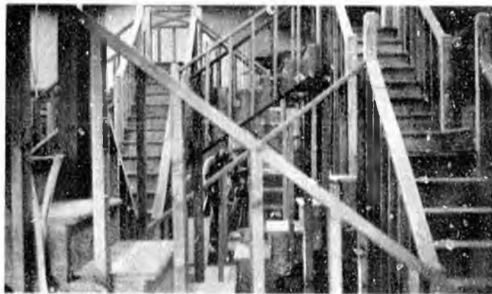
This stair project is an example of work performed by Apprentices in this Program.
