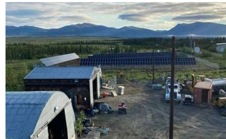
Shungnak-Kobuk Community Solar Independent Power Producer. Photo Credit: U.S. Department of Energy.
