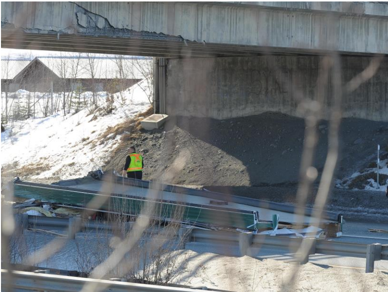
Aftermath of truck collision with Glenn Hwy. bridge in 2018. Photo from Anchorage Daily News
